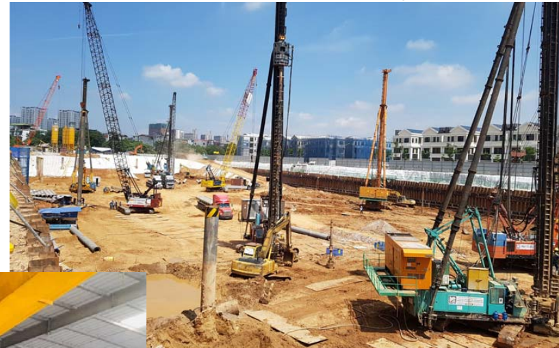
The first project in Hanoi capital to apply the pre-boring method
